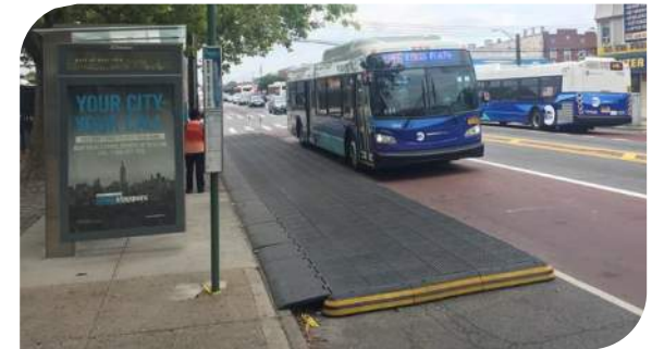
Above Top: The City of Fremont has used a combination of painted bulb outs with self-watering landscape planters to achieve this effect. Above: Prefabricated boarding islands or parklet-style boarding islands can be used to extend the sidewalk and allow buses to stop in line to improve transit reliability. Photo credit: www.zicla.com
