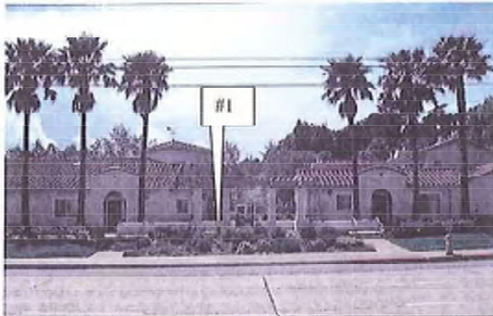
87. FRONT VIEW OF CREEKSIDE VILLAS
