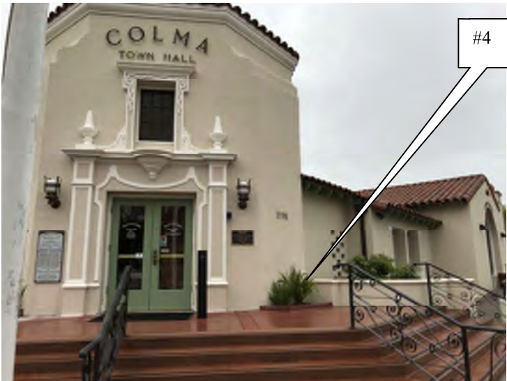
78. Typical planters along Town Hall Frontage.
