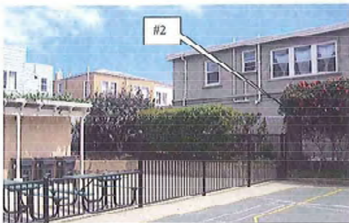
101. AREA TO THE RIGHT OF THE OUTSIDE STORAGE BUILDING
