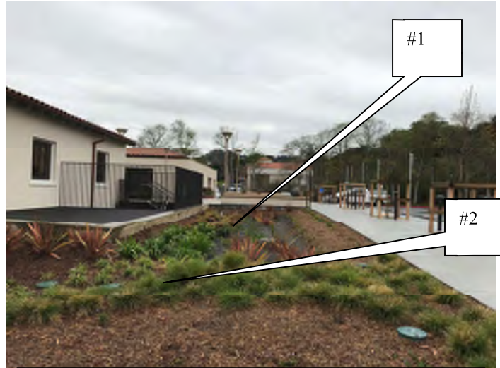
75A. Bio-Retention area looking towards Town Hall from ECR
