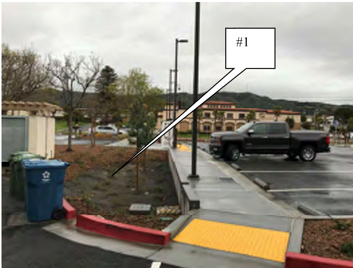
75. Bio-Retention area in the Town Hall Parking Lot
