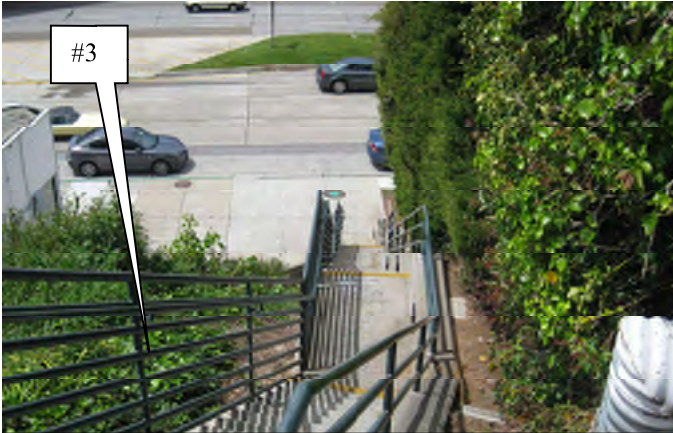
63. E STREET STAIRS LEADING TO EL CAMINO REAL
