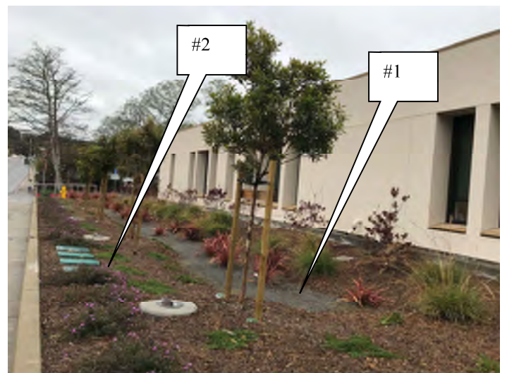
75C. Bio-Retention area along Serramonte Blvd.
