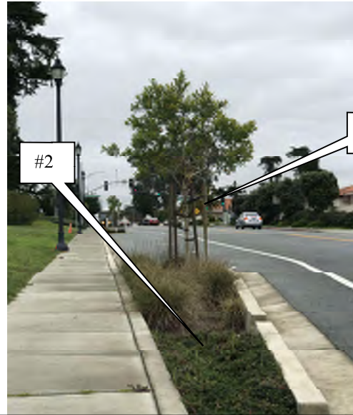
71. HILLSIDE BOULEVARD NEAR SERRAMONTE BLVD.
