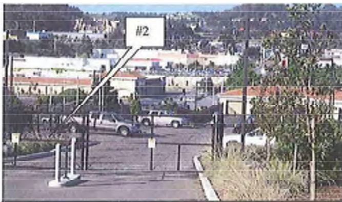
83. COLMA POLICE FACILITY VIEWING WEST AT SERRAMONTE DRIVEWAY
