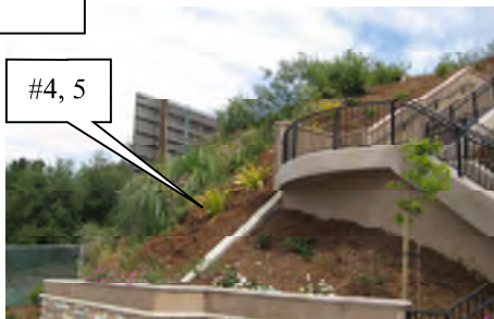
59. D STREET STAIRS
