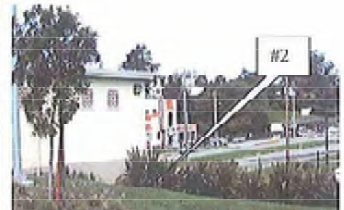
86. REAR PARKING LOT OF THE COLMA POLICE FACILITY
