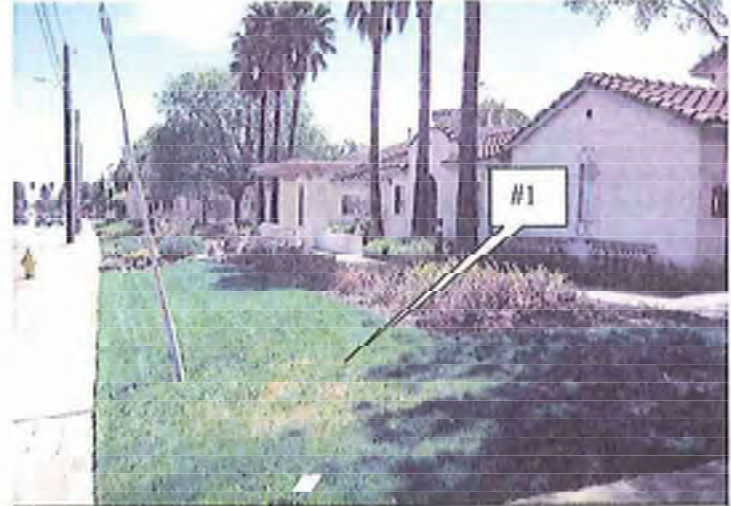
88. FRONT VIEW OF CREEKSIDE VILLAS
