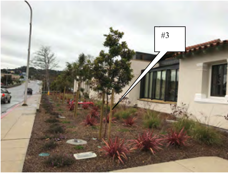
77. Town Hall frontage along Serramonte Blvd
