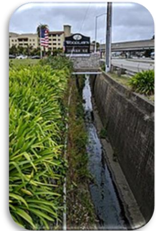
Colma Creek: from the west side of El Camino Real along Woodlawn Memorial Park
