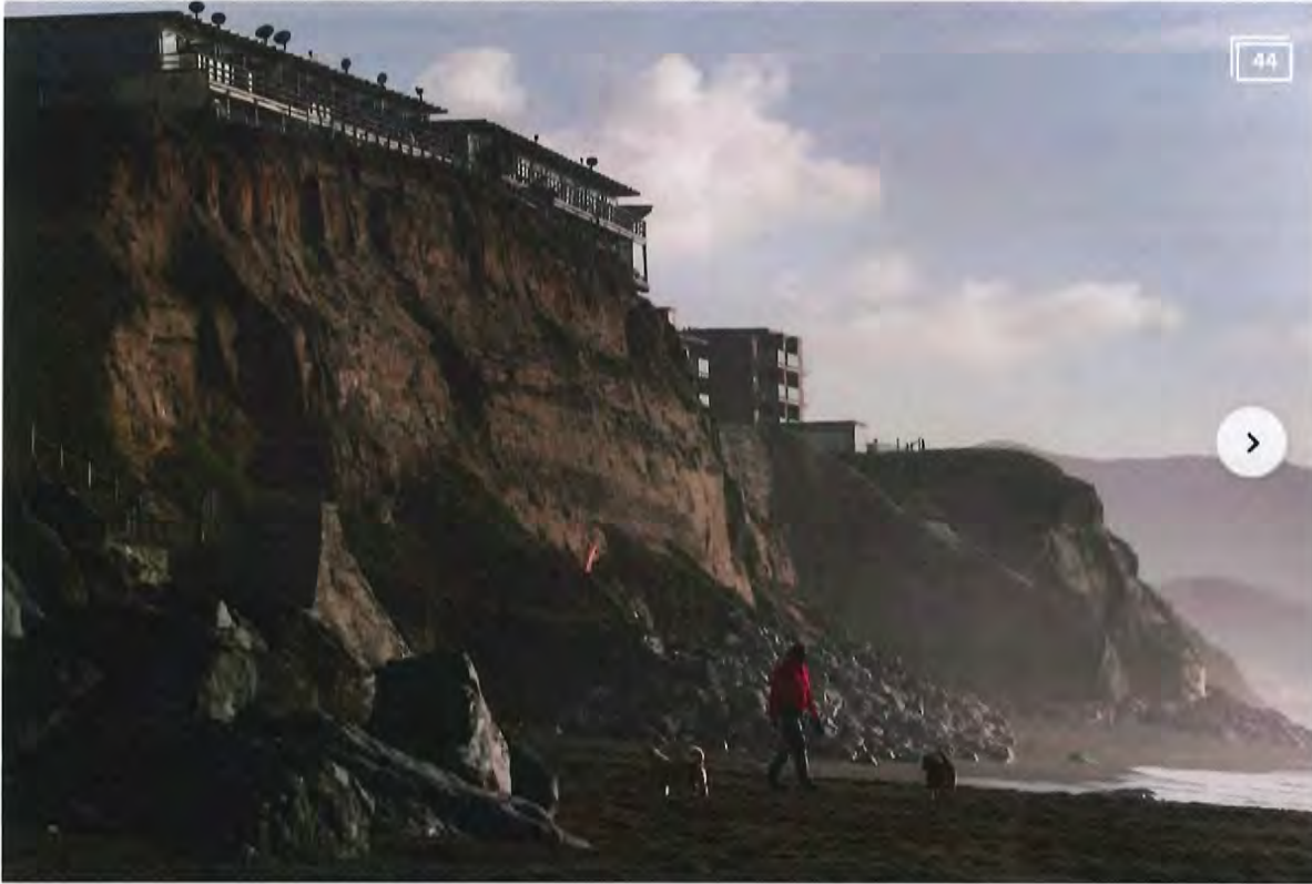
Properties along Esplanade Ave can be seen perched on the edge of an eroding cliff Dec. 23, 2015, in Pacifica, Calif. The center property is vacant. (Leah Millis/San Francisco Chronicle)
