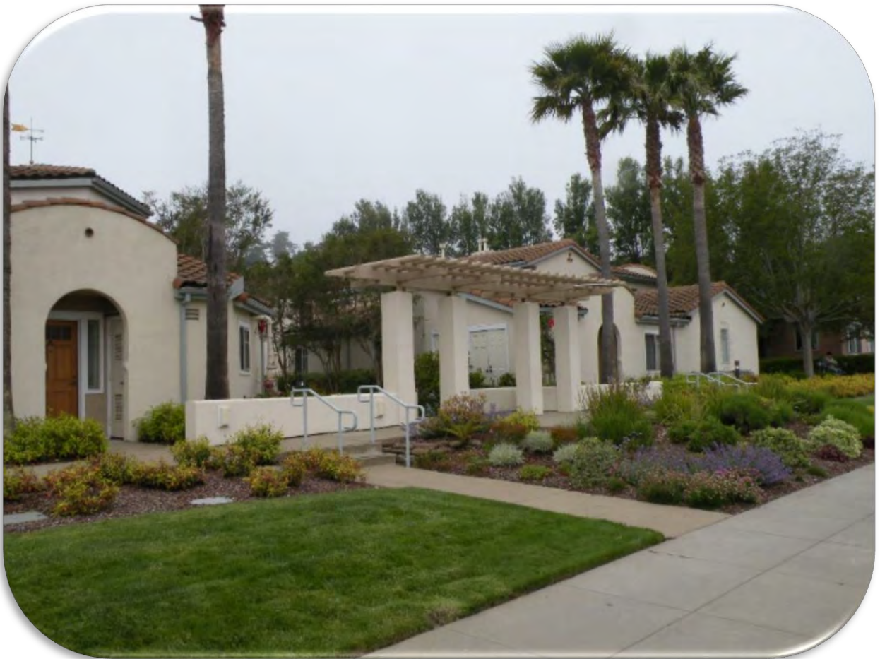
The Town of Colma owns 18 Senior Housing Units, located on El Camino Real
