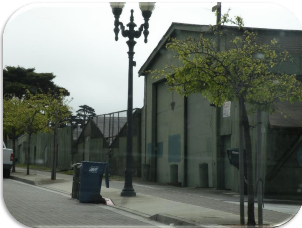
This former greenhouse is located in Sterling Park. The parcel is zoned for residential use and has a realistic development potential of nine single family detached units.
