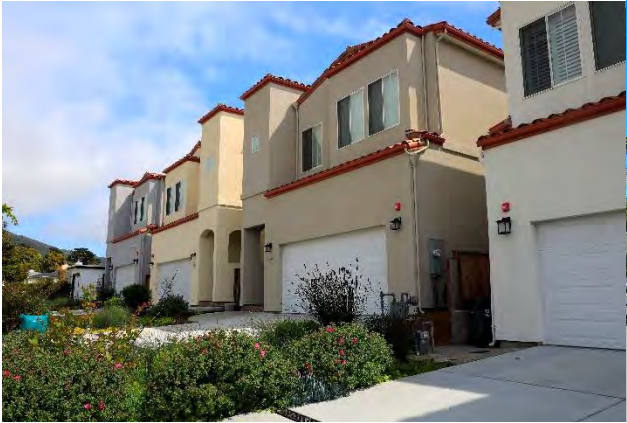
Single Family Residential Homes on B Street
