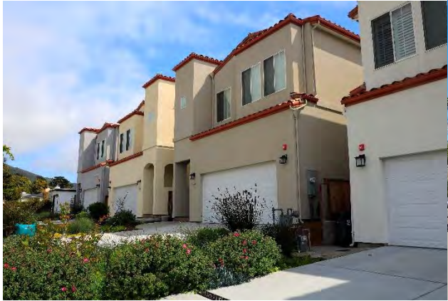
Single Family Residential Homes on B Street
