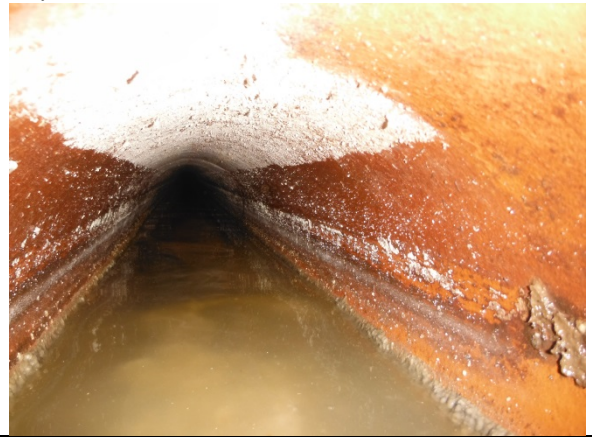
Inlet Pipe: P1
