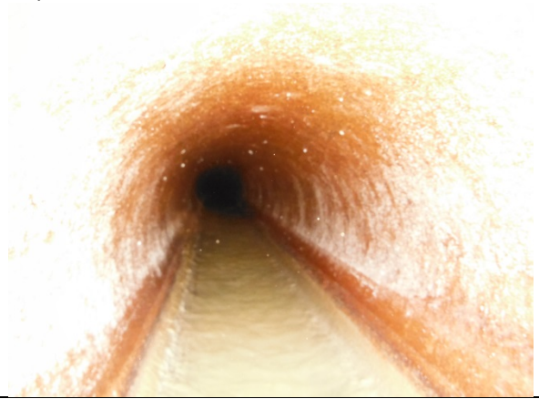
Inlet Pipe: P1
