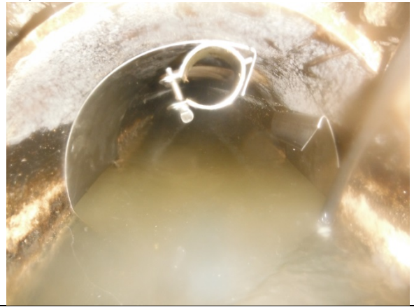
Inlet Pipe: P1
