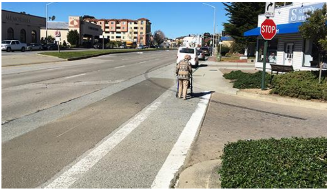
Non-Compliance curb ramp by El Camino Real/F Street Intersection used by people of disabilities
