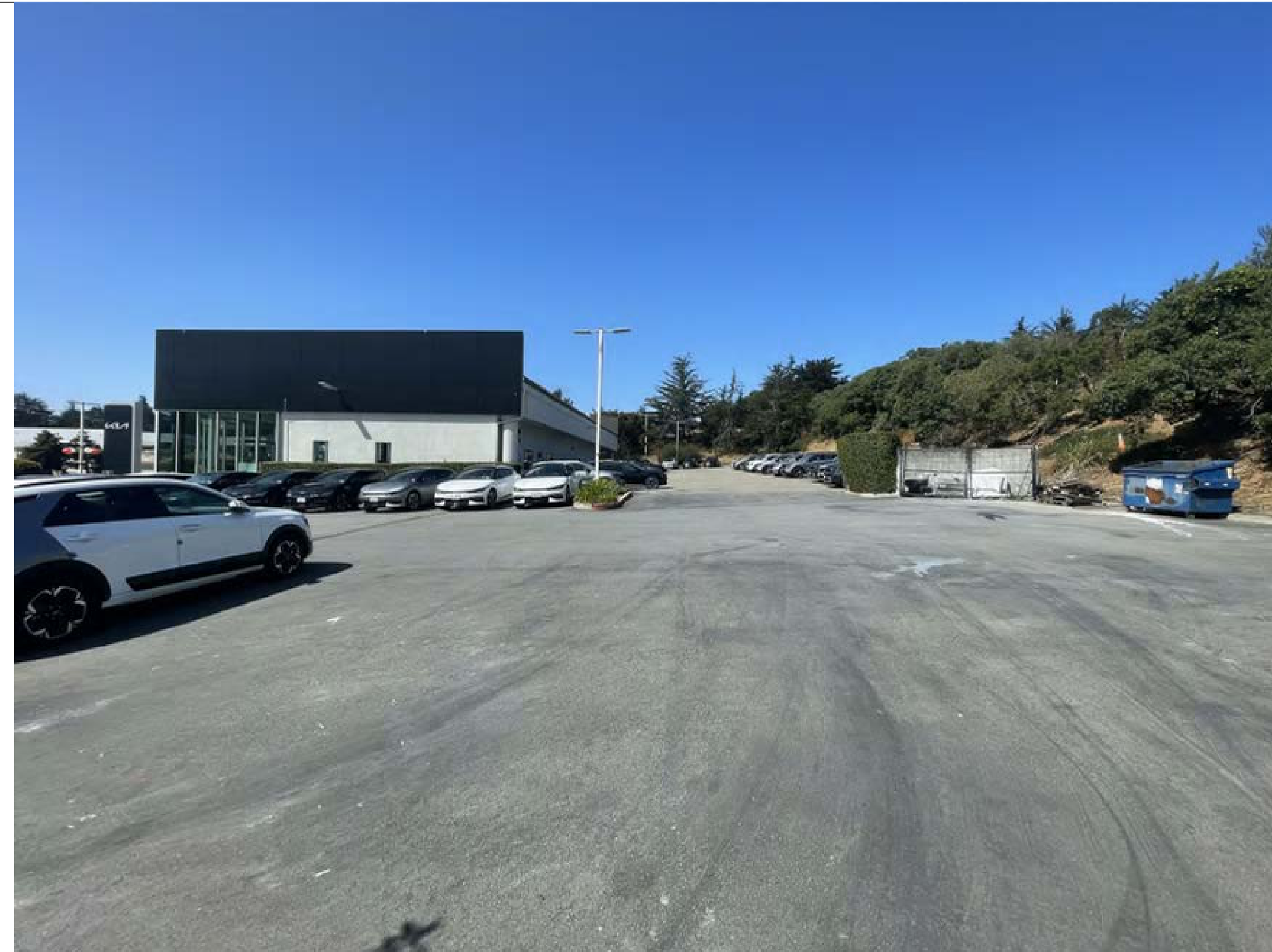
PROJECT PROPERTY (E) NORTH REAR DRIVE AISLE 4
