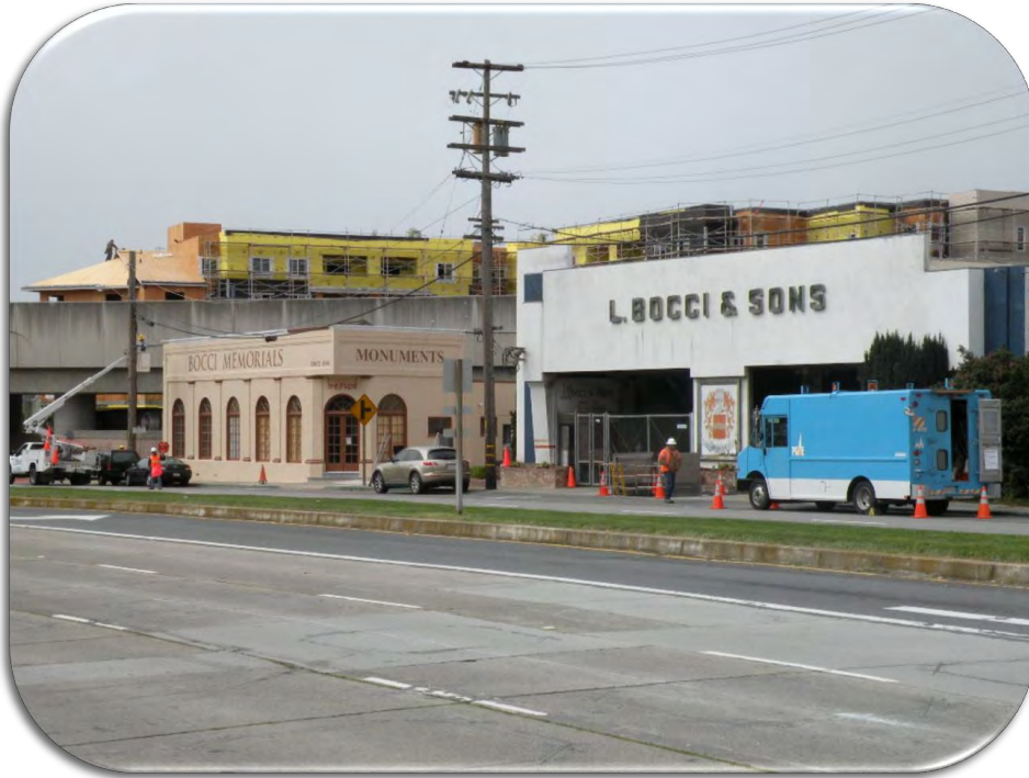
The 0.6-acre Bocci site at 7778 El Camino Real has a realistic development potential of 24 high density multi-family units. Site specific constraints on the property include a utility easement serving the adjacent Colma BART Station.
