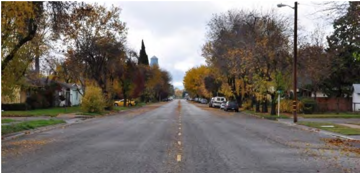
A typical local road in Corning
