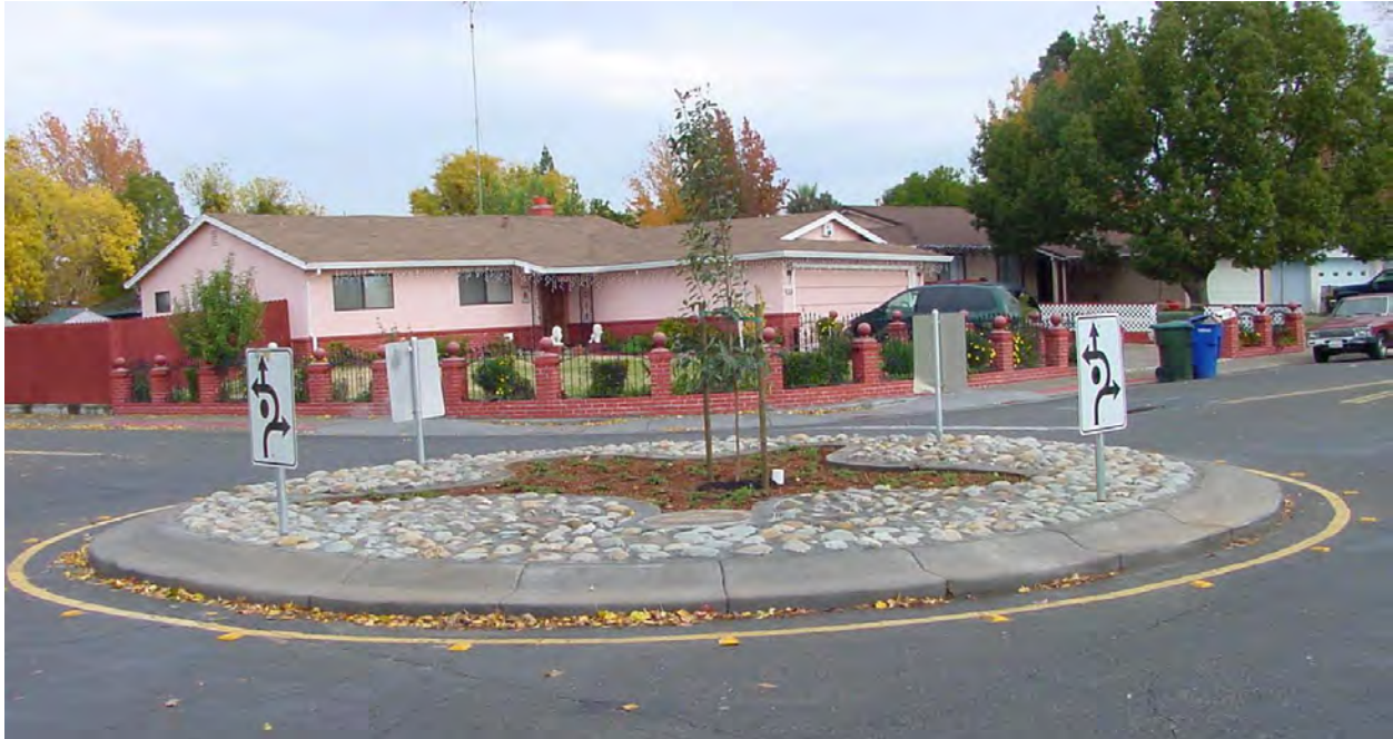
Example of a central island of a roundabout in a neighborhood context
