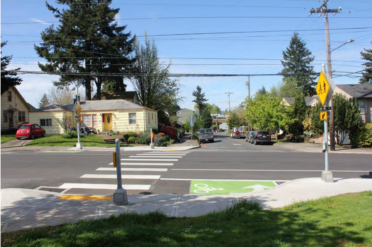
Example of enhanced pedestrian crossing
