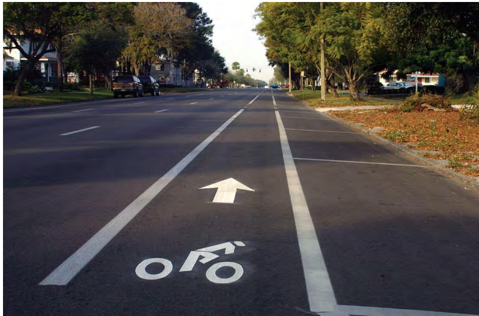
Example of a Class II Bike Lane with on-street parking
