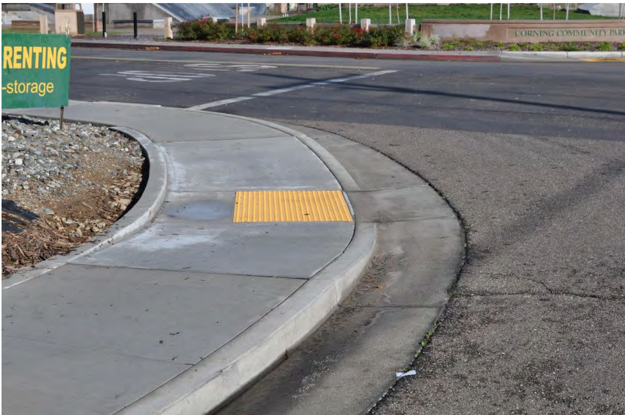
Pedestrian curb ramp compliant with Americans with Disabilities Act (ADA)
