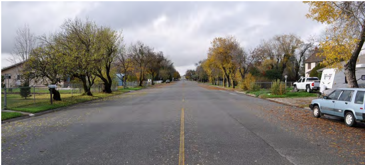
Typical Corning Street with a greater than 50' curb-to-curb distance
