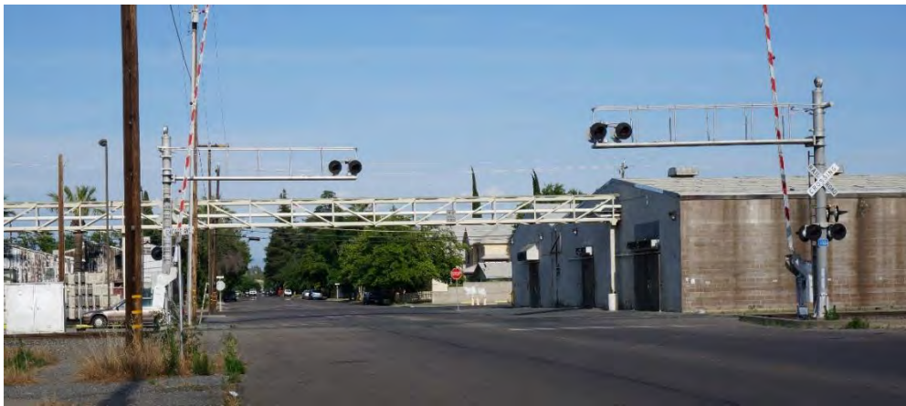
Existing railroad crossing at South Street
