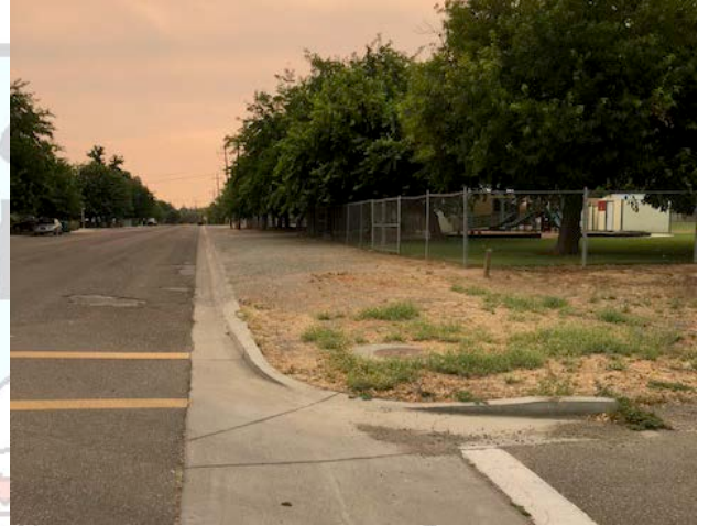
Missing Sidewalk at Southeast corner of Pear Street Intersection
