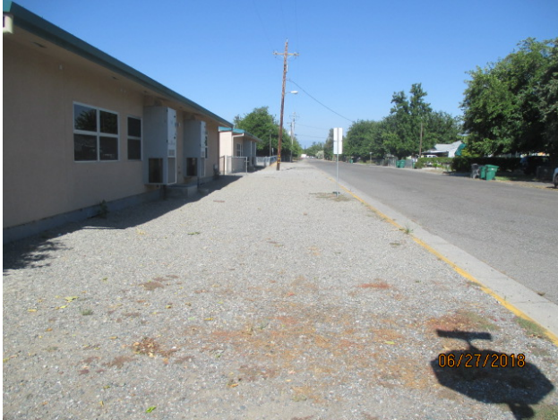
Missing Southerly Sidewalk looking West on Almond Street
