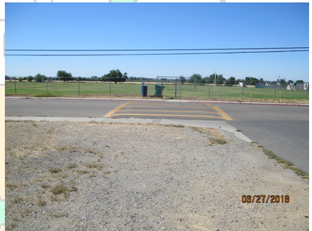
Missing Sidewalk Connection on Pear Street at Fig Lane
