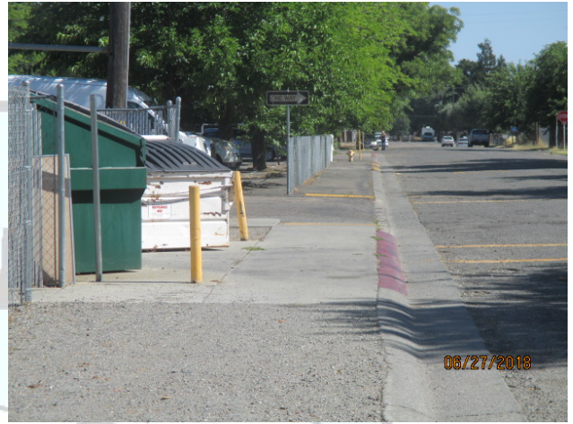
Missing Sidewalk South of Hickory Street Intersection
