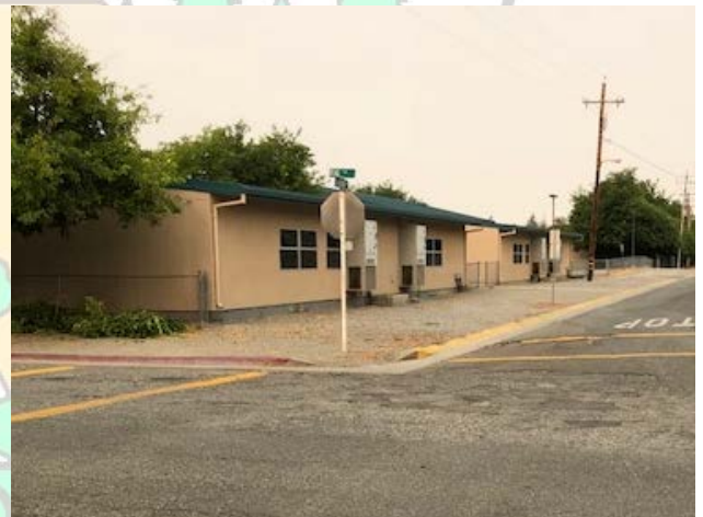
Missing Sidewalk and Pedestrian Ramp on Southwest corner of Almond Street Intersection
