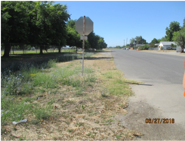
Missing Sidewalk on East Side of Pear Street
