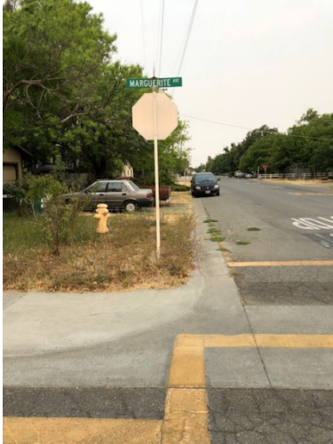
Missing Sidewalk on Almond Street between Fig Street and Marguerite Ave
