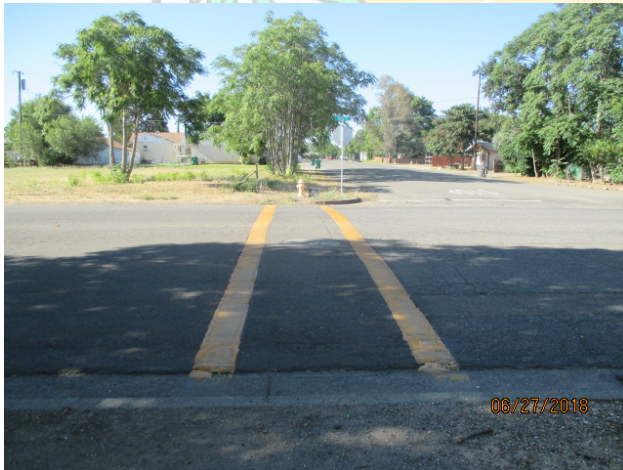
Existing Crosswalk and Missing Pedestrian Ramp at Intersection
