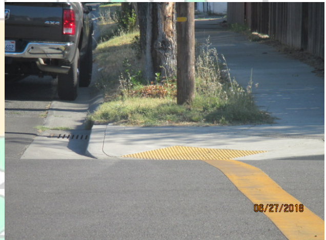
Inadequate Pedestrian Ramp on Northeast Corner of Intersection
