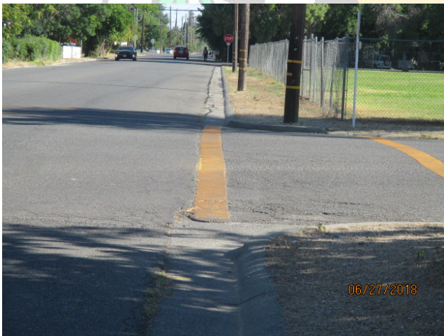
Existing Crosswalk and Missing Pedestrian Ramp on East Side of Intersection
