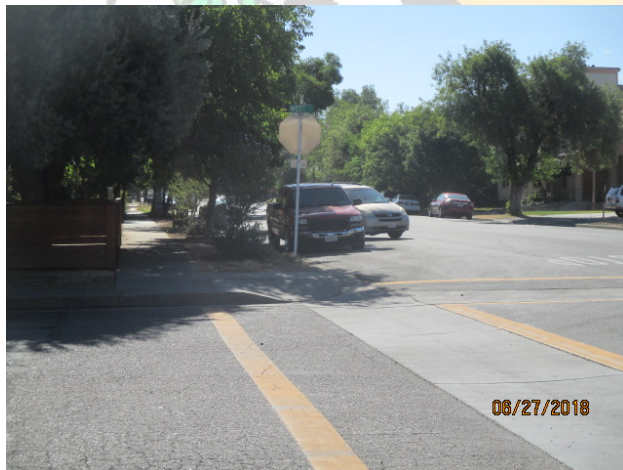
Existing Crosswalk and Inadequate Pedestrian Ramp at Northeast Corner of Intersection
