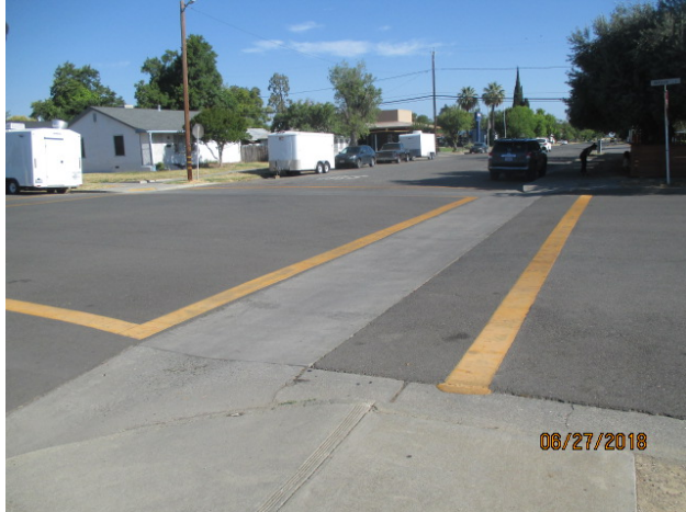
Existing Crosswalk and Inadequate Pedestrian Ramp at Southeast Corner of Intersection
