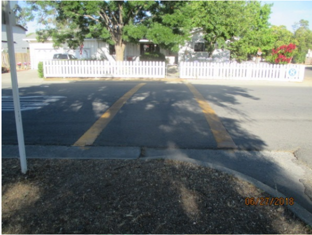
Existing Crosswalk and Missing Pedestrian Ramp on South Side of Intersection
