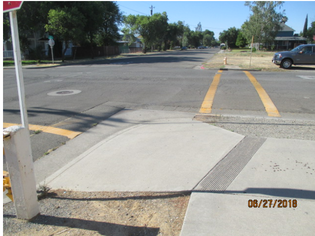
Existing Crosswalk and Inadequate Pedestrian Ramp at Northwest Corner of Intersection
