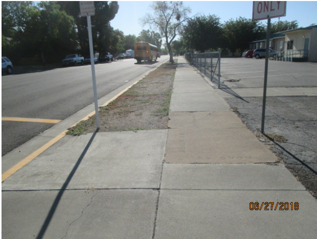
Existing Sidewalk and Missing Pedestrian Ramp on South Side of Marin Street
