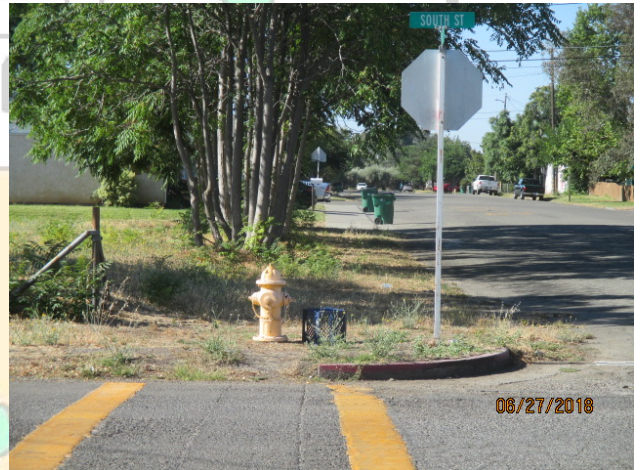
Existing Crosswalk, Missing Sidewalk, and Missing Pedestrian Ramp at Intersection
