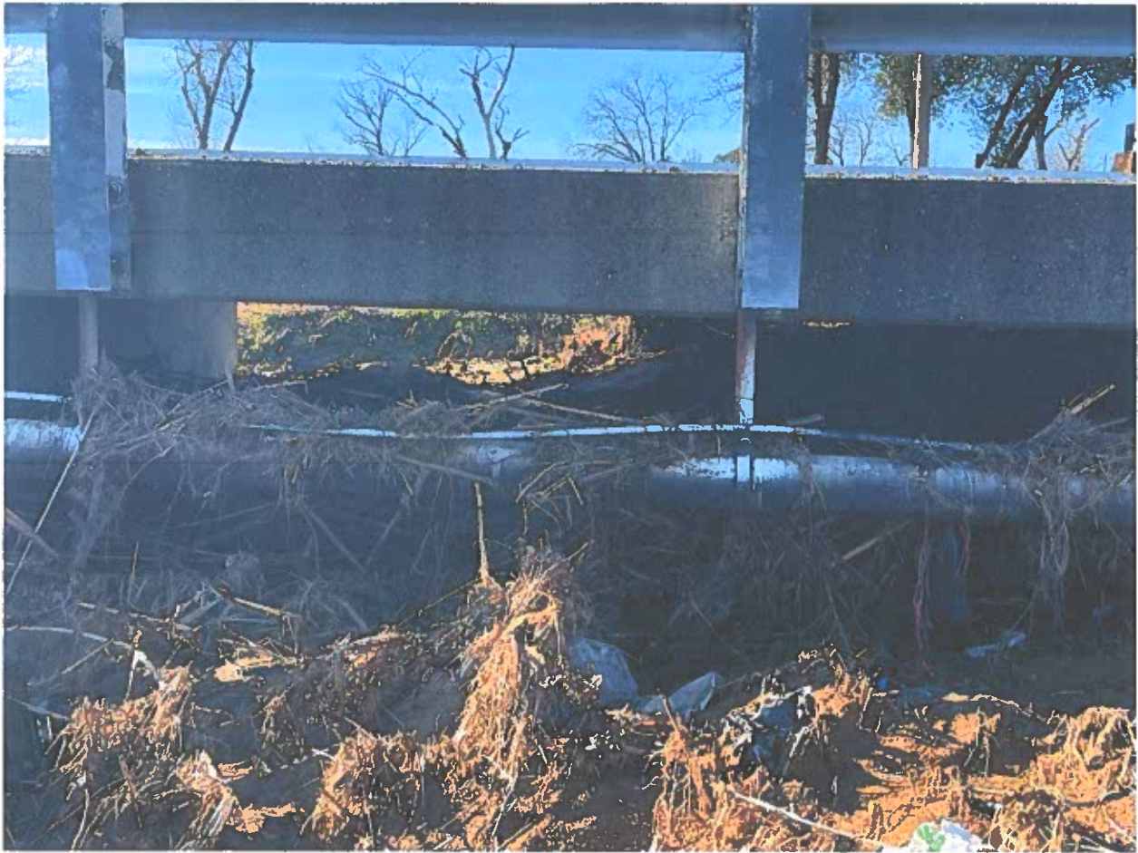
Burch Creek Bridge at eastside of Highway 99W
