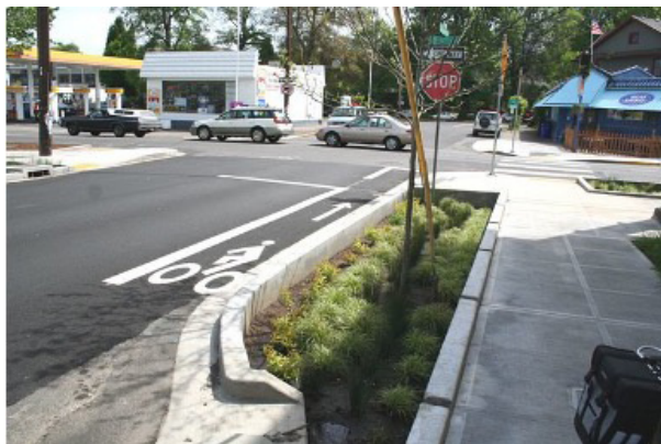
Figure 4. Bioswales with drought tolerant plants help to reduce stormwater runoff, filter pollution, and provide cooling benefits to the surrounding area
