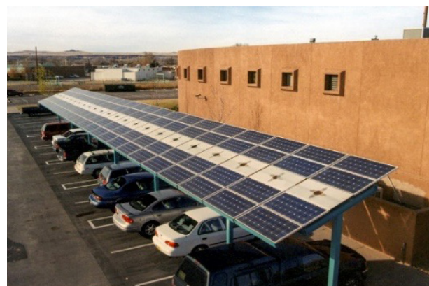
Figure 5. Solar photovoltaic carports help to keep parking lots cool while also generating renewable energy
