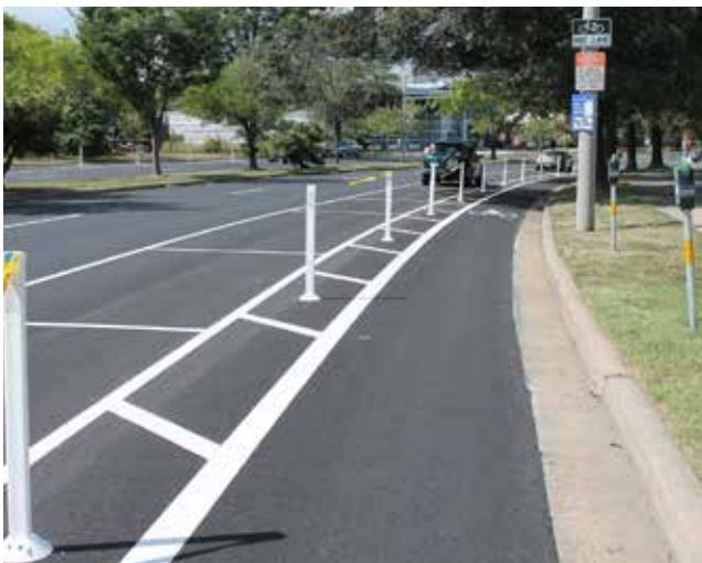
Cycle Track with Safety Bollards
