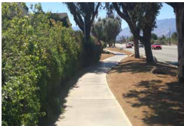
Arterial sidewalk along Palm Drive south of Camino Campanero
