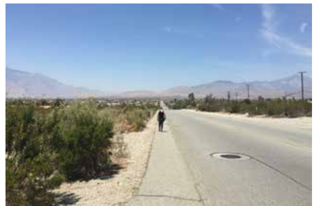
Sidewalks on Hacienda Avenue and Verbena Drive
