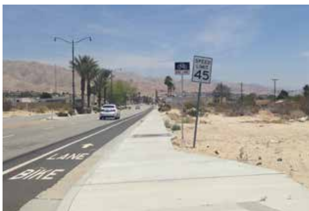
Arterial sidewalk on Pierson Avenue by Desert Hot Springs High School
