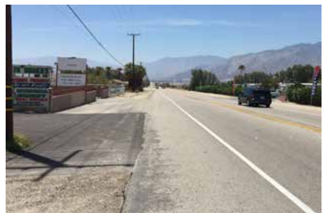
Lack of sidewalks on Indian Canyon Drive
