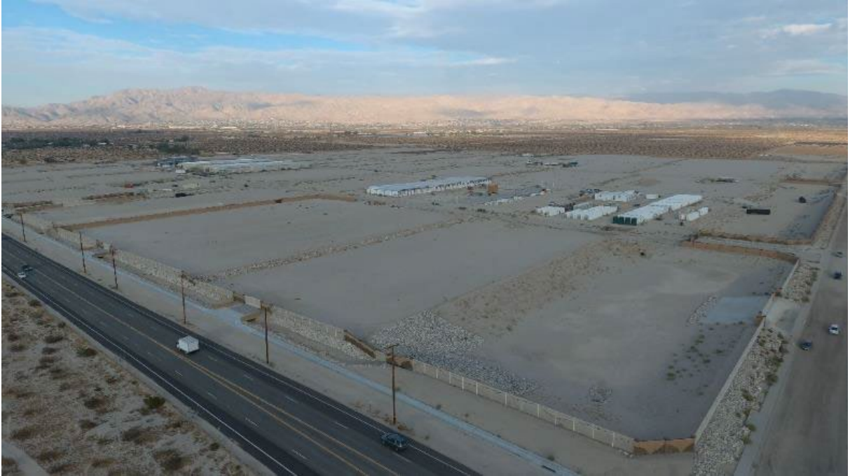
Photo 1 View Looking Northeast at 19th Avenue and Indian Canyon Drive Intersection. Parcels 101, 31, and 30 in Foreground (right to left). Rough Grading Completed (November 2020)
