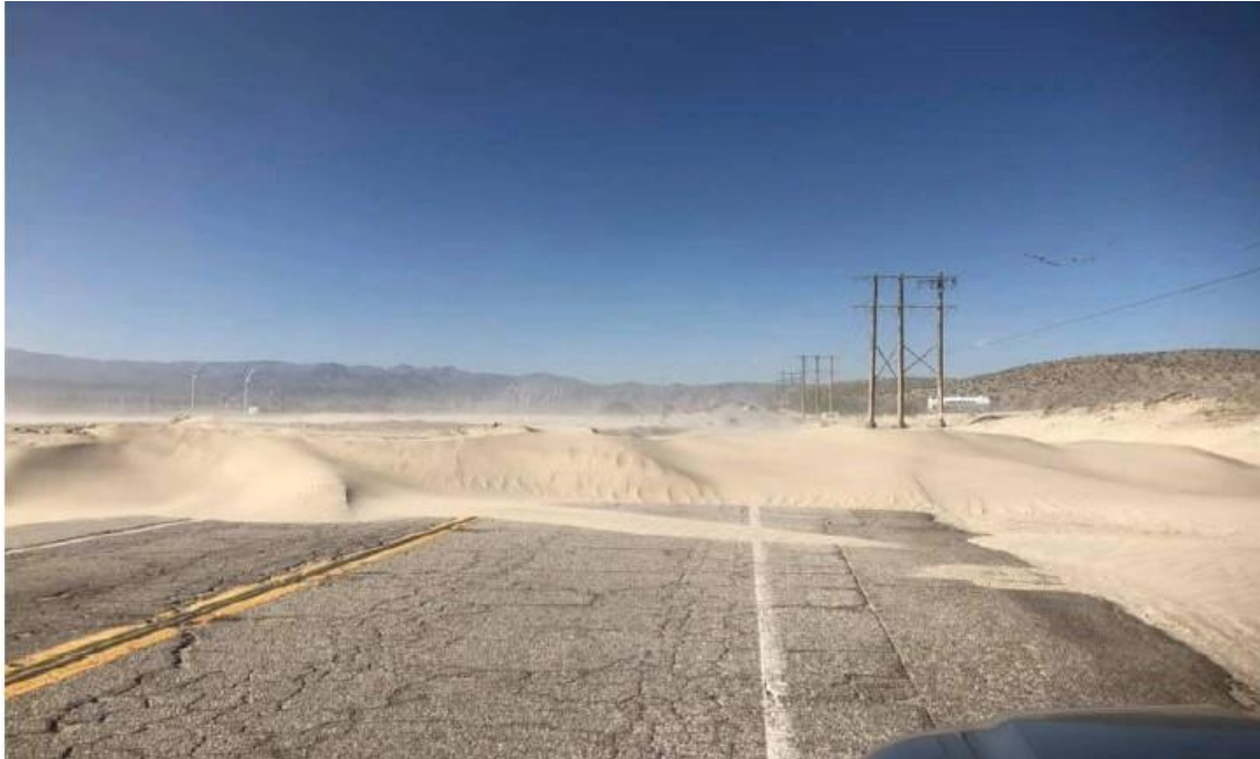
FIGURE 1-3: NORTH INDIAN CANYON DRIVE (SEDIMENT DEPOSITS)
