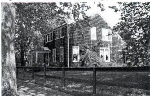
Fig. 16. Osborn House, 88 Newtown Lane
