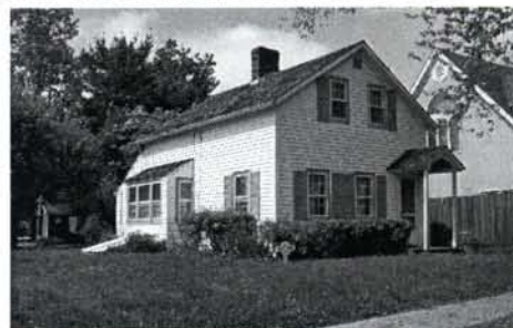
Fig. 17. Muchmore House, 83 Newtown Lane
