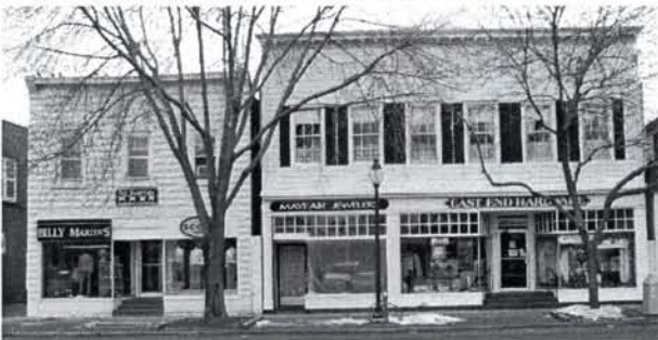
Fig. 3. Northrup Building and A.O. Jones Building, 47 and 51 Newtown Lane
