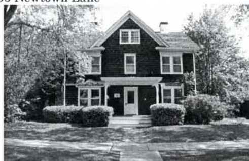
Fig. 15. Filer House, 98 Newtown Lane
