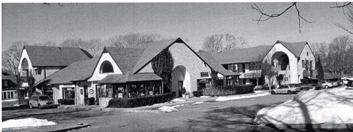
Fig. 24. Red Horse complex, 74 Montauk Highway
