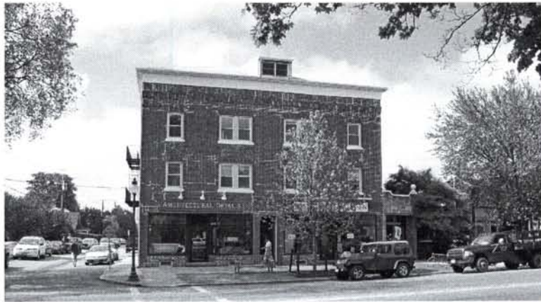
Fig. 18. Cavagnaro Building, 105 – 107 Newtown Lane
