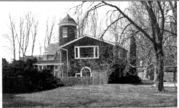
Herrick Carriage House & Windpump Tower, 1888 Isaac Henry Green Jr., architect
