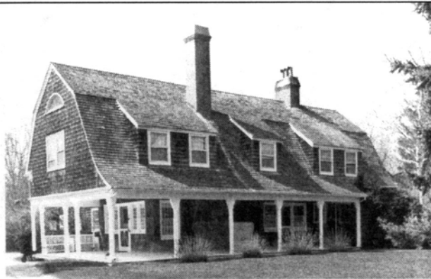
George E. Munroe House, 1889 Isaac Henry Green Jr., architect
