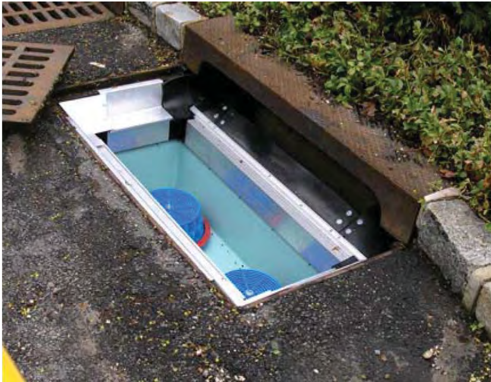
Figure C-1 StormBasin Catch Basin Insert - Clean
