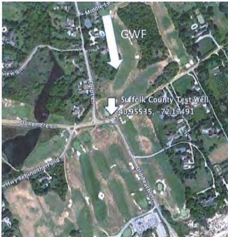
Figure 12 - SCDHS Monitoring Well Location
