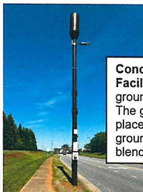
(6) Concealed Small Cell Towers/Poles
