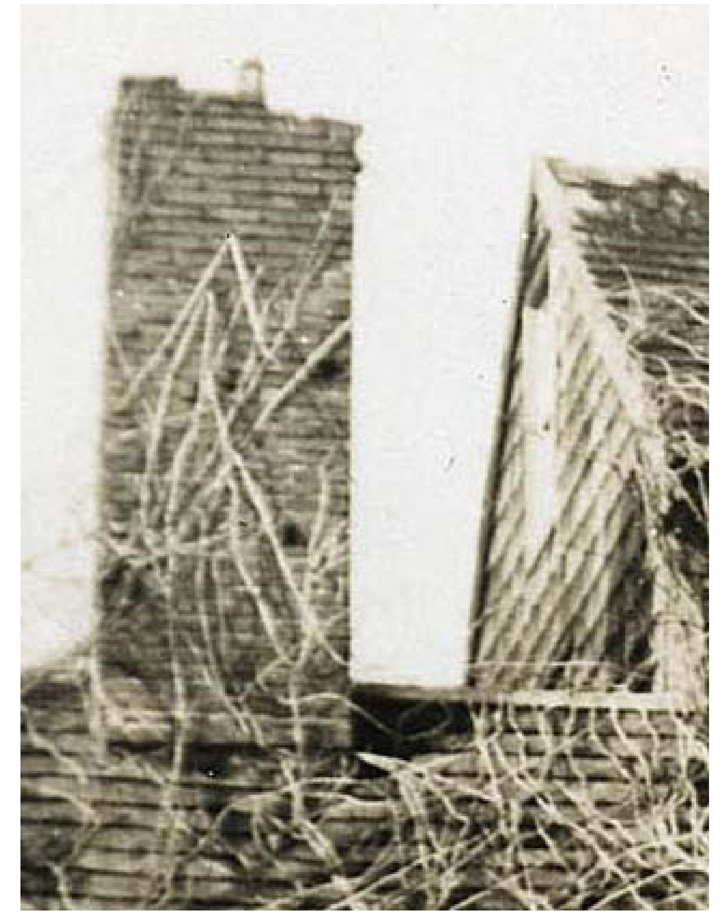
VIEW OF CLOCK SHOP CHIMNEY SHOWING PROJECTING COURSE AT ROOF SHINGLES AND BRICK SEPARATING FORGE AND FIREPLACE FLUES c. 1940 photo, East Hampton Historical Society.
