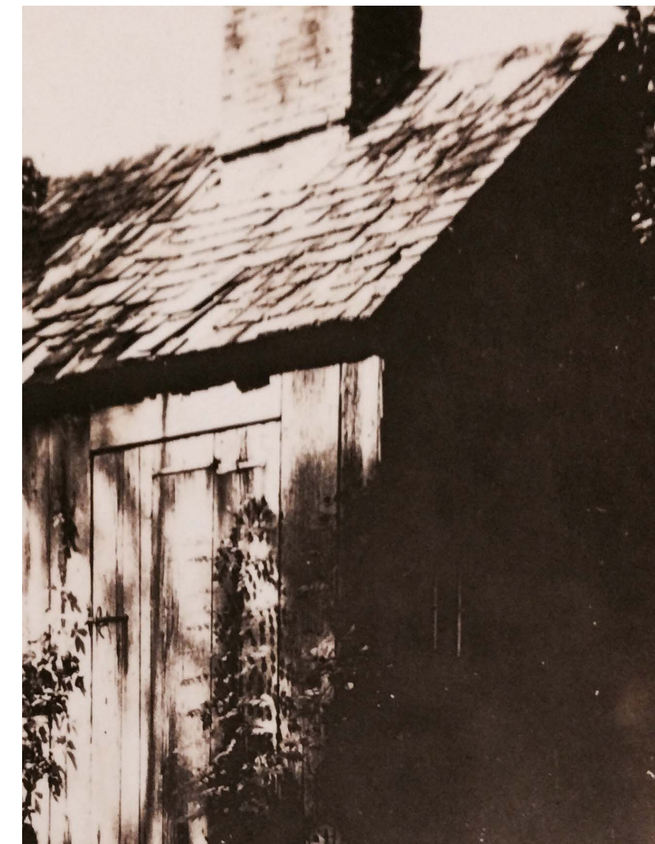
VIEW OF EAST WALL OF CLOCK SHOP SHOWING CHIMNEY AND PROJECTING COURSE AT ROOF SHINGLES Eugene Amrbruster photo, c. 1923, New York Historical Society.
