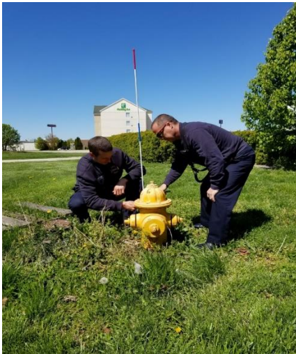
Fire Department personnel placed over 500 hydrant markers across the City providing firefighters with an improved method for spotting fire hydrants, especially under low-light and bad weather conditions.
