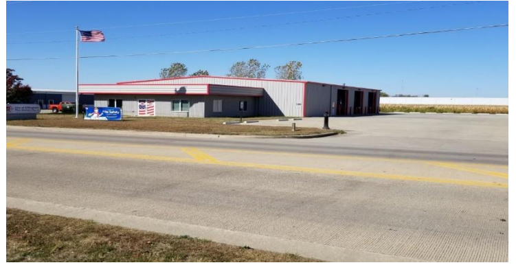
The Fire Department moved into the new Fire Station 2 located at 500 W Jaycee Ave. The existing building was repurposed – saving the City and taxpayers about 1.7 million dollars versus constructing the building new from the ground up. The new station provides safer and faster response times.
