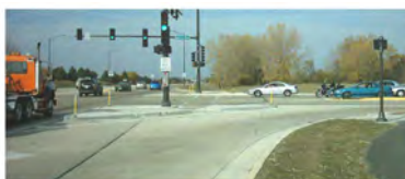
Figure 12 Intersection design methods to reduce sidepath conflicts. Top left: bringing crossing closer. Top right: warning signage. Bottom left: right-turn refuge islands.
