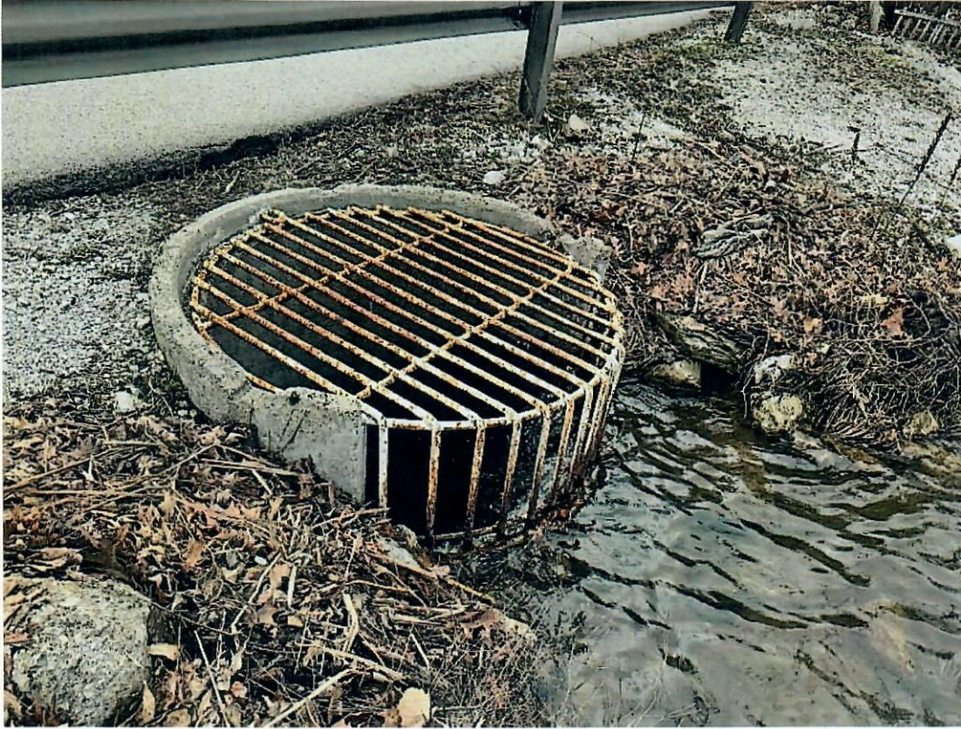
Drop Manhole Control Structure- 3/27/24
