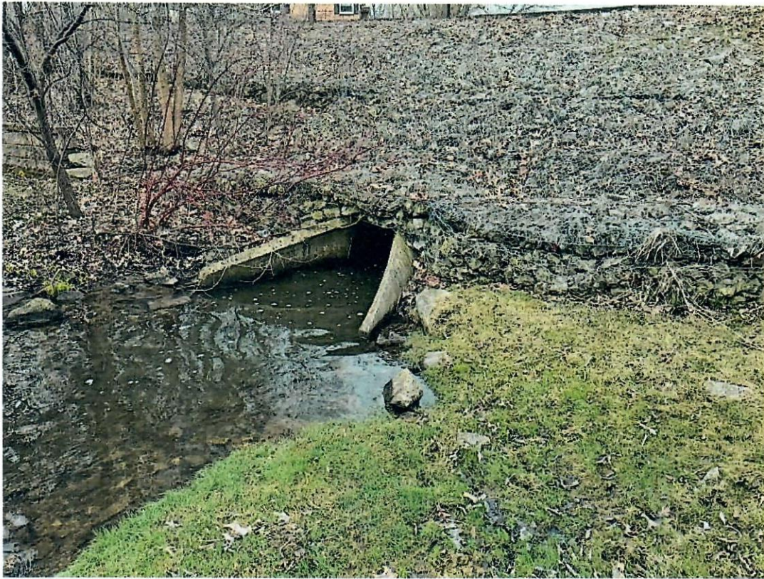
36" RCP Outlet Pipe- 3/27/24
