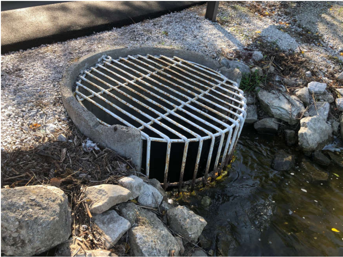
Drop Manhole Control Structure- 9/30/20
