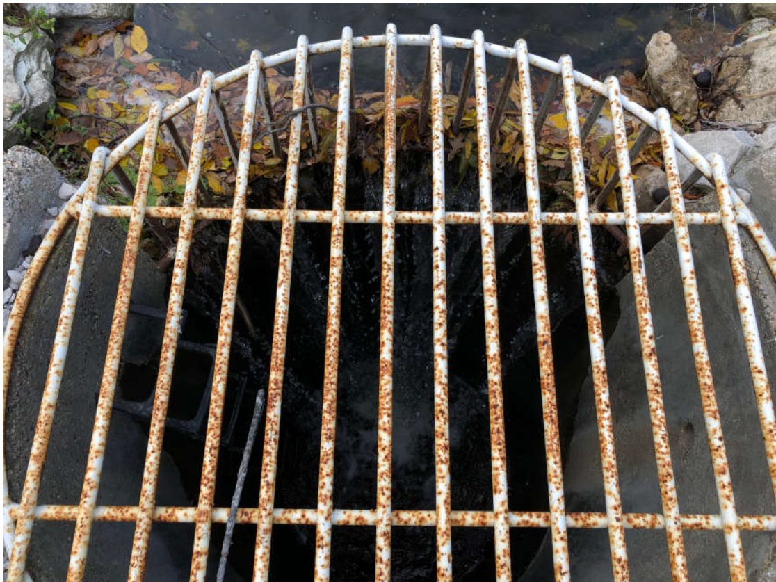
Control Structure- Water Level Approximately 10" Above Concrete Sill- 11/1/2021
