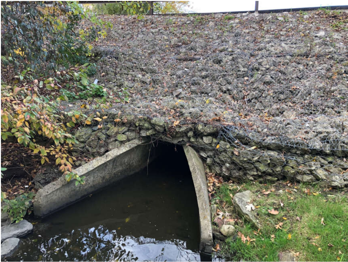
36" RCP Outlet Pipe- 11/1/2021
