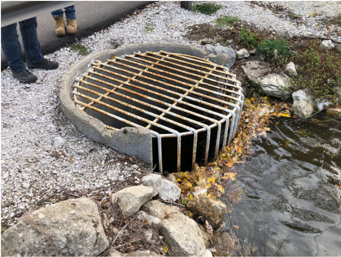
Drop Manhole Control Structure- 11/1/2021
