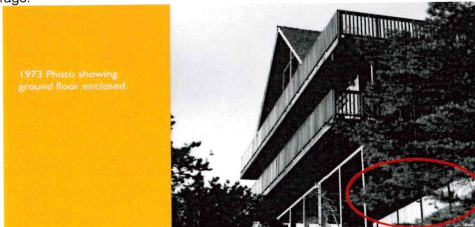
Figure 1. Existing Ground Floor Condition
