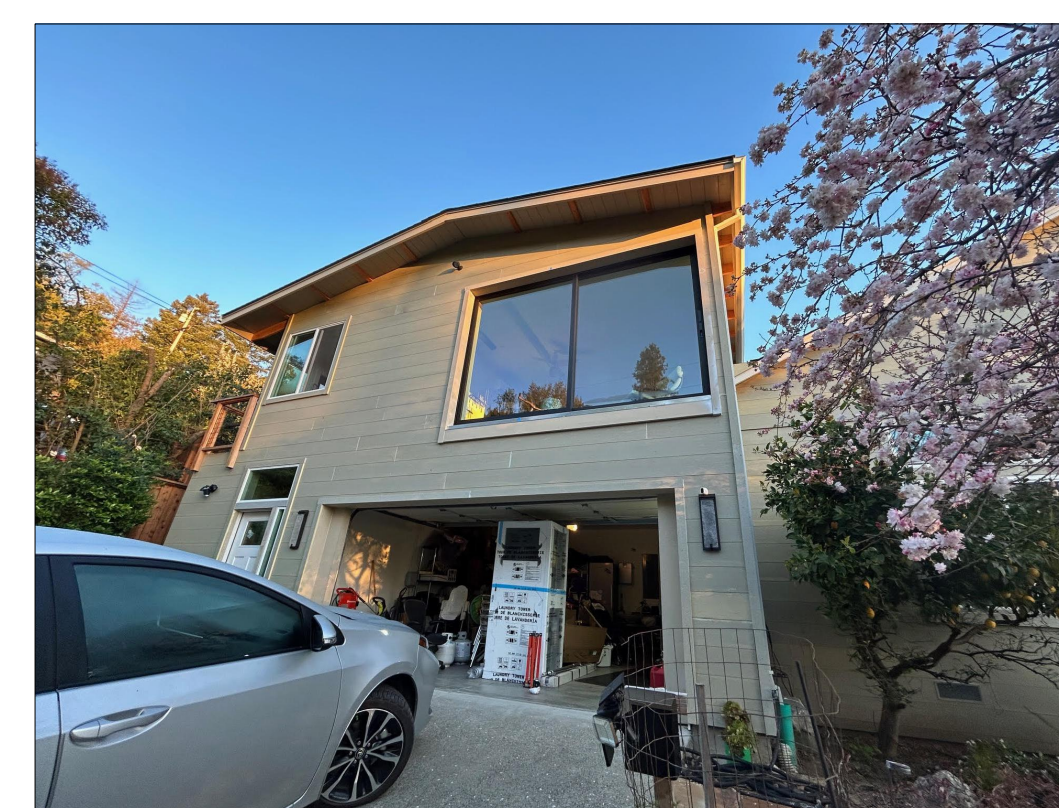
FRONT OF ADU AND GARAGE
