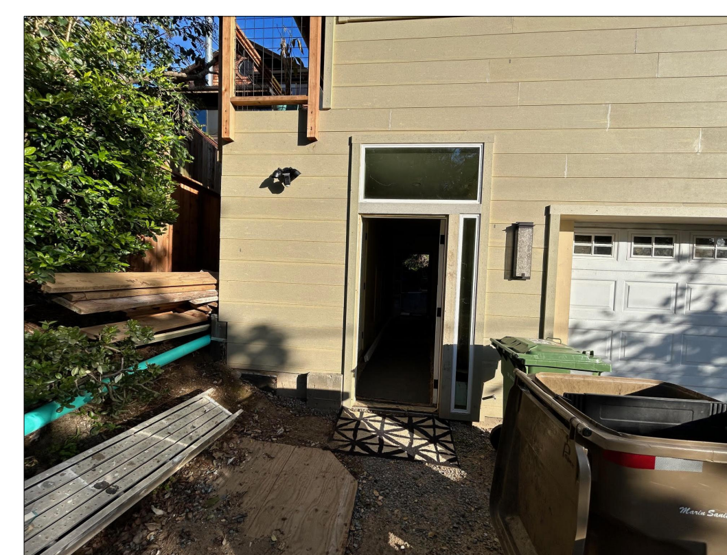
UNDER ADU AND STAIR AT FRONT
