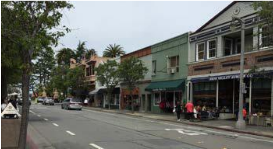
Façade: Before Renovation
