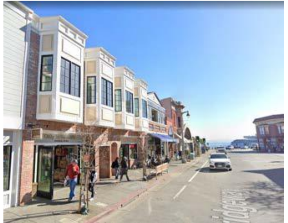
Current Built Conditions after Renovation
