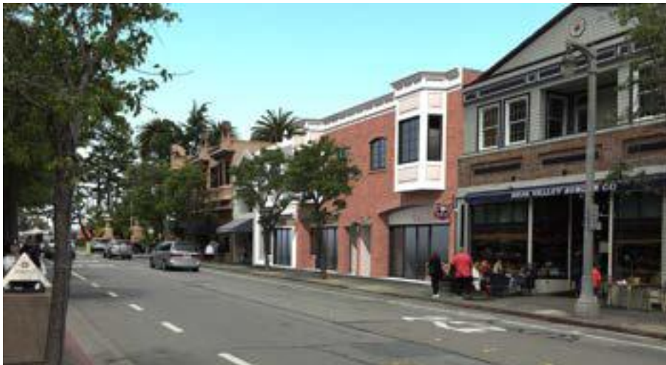
Façade: After Renovation
