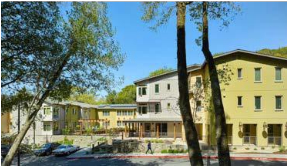
View of Existing Building from Street
