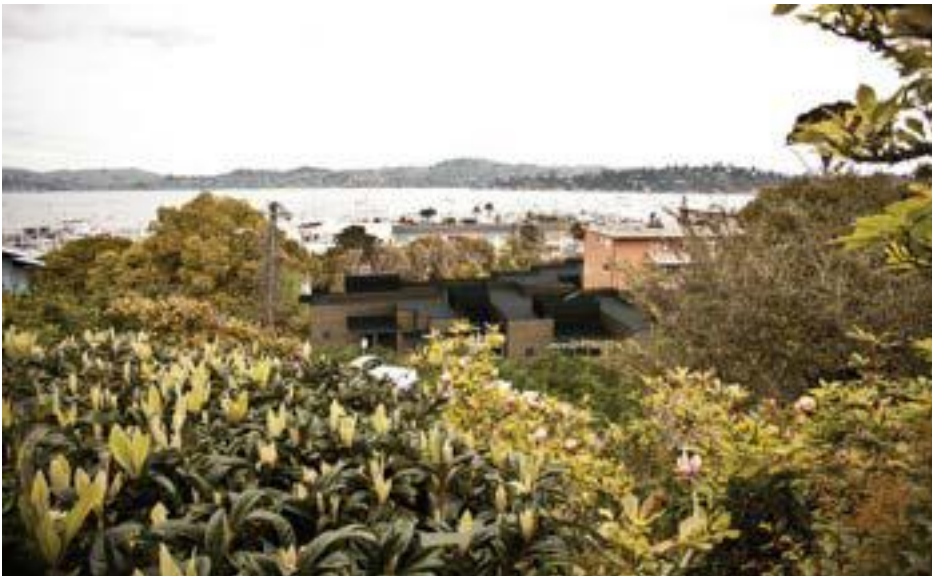
View over Project after Construction
