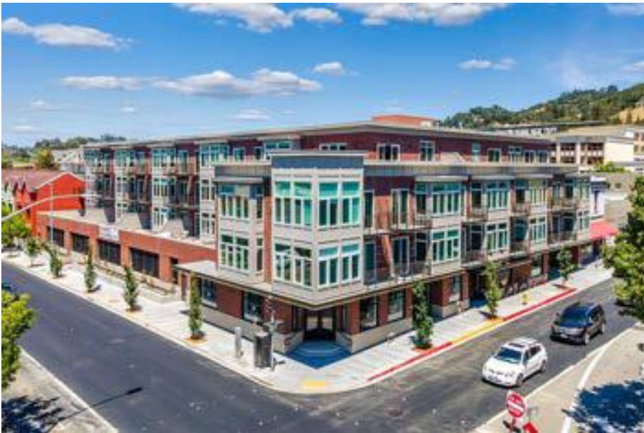
Existing Building Facade
