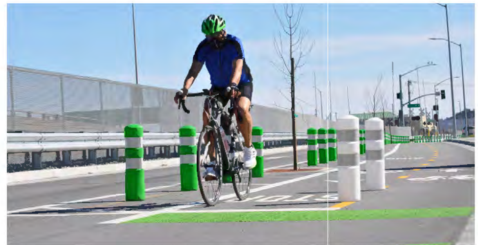
Recent improvements on Francisco Boulevard West increase safety and comfort for cyclists.
