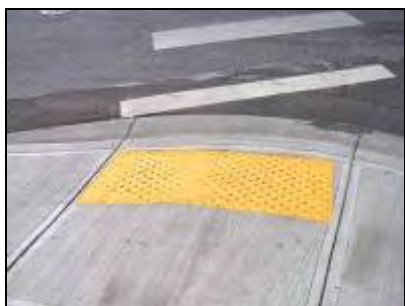
A curb ramp with truncated domes
