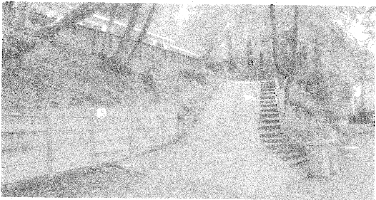
Trees 1, 2, 3 & 4 have been employed as retaining wall supports which threatens both the trees and the walls.
