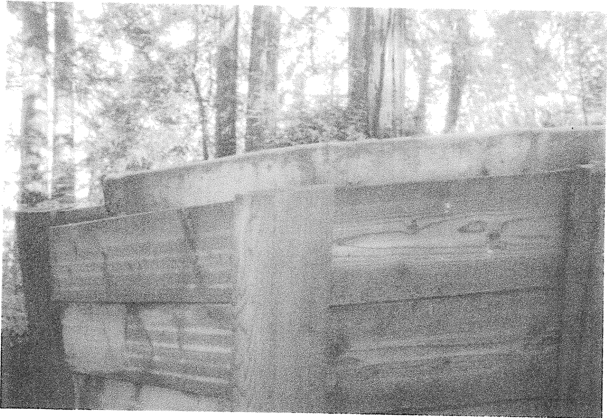
The failing retaining wall above Trees #5 and 6. Failure of the wall and fill soil will impact Trees #5 and 6.
