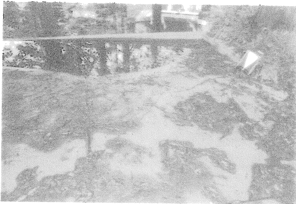
The failing parking turnout. Tree #1 is shown in the upper right hand corner just 5" from the slab. Tree #1
