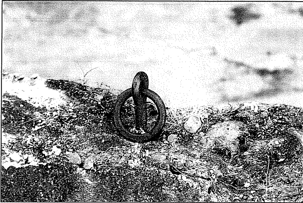
Figure 11: Example of hitching ring on concrete wall along north façade
