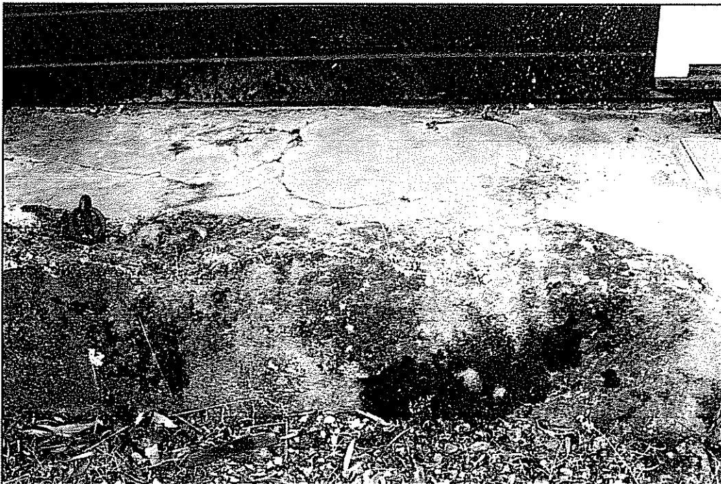
Figure 10: Concrete wall along north facade
