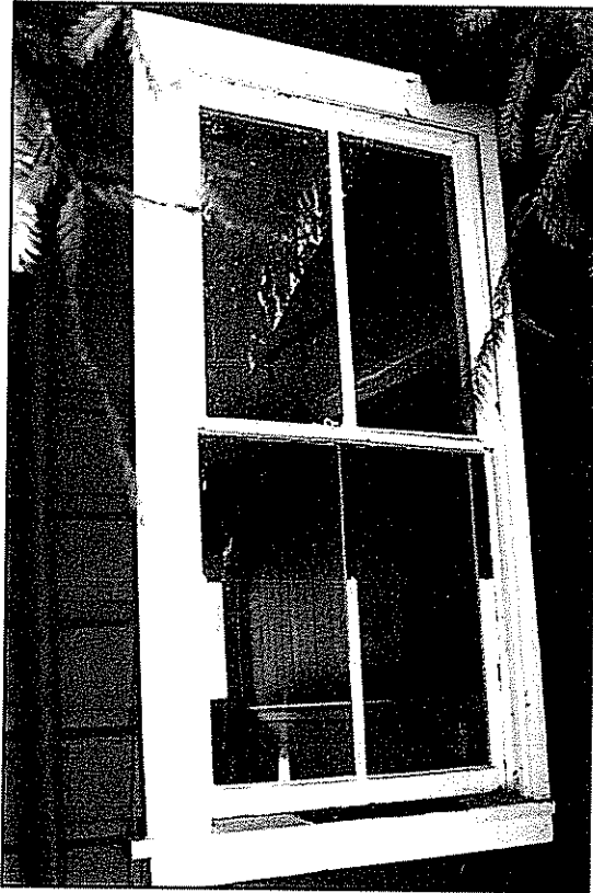
Figure 20: South elevation, window at southwest corner
