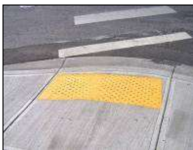
A curb ramp with truncated domes
