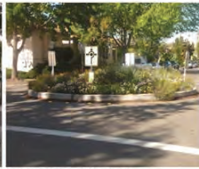
potential traffic circle
