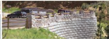
retaining walls to add parking
