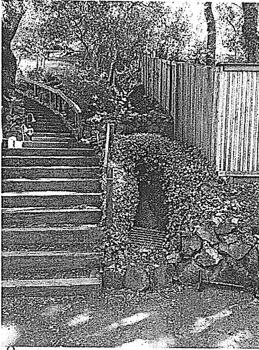
Figure 3 Existing Drainage Improvements
