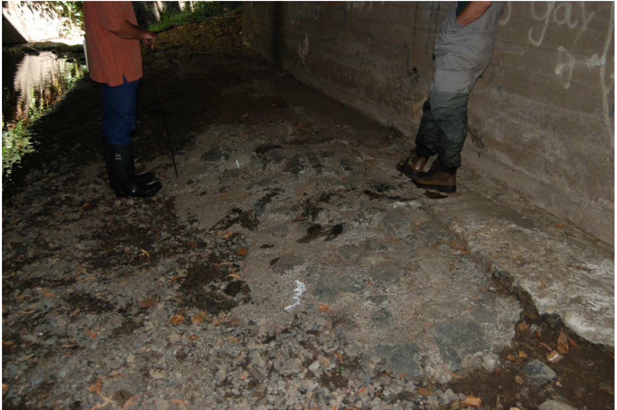
Exposed bedrock under the bridge
