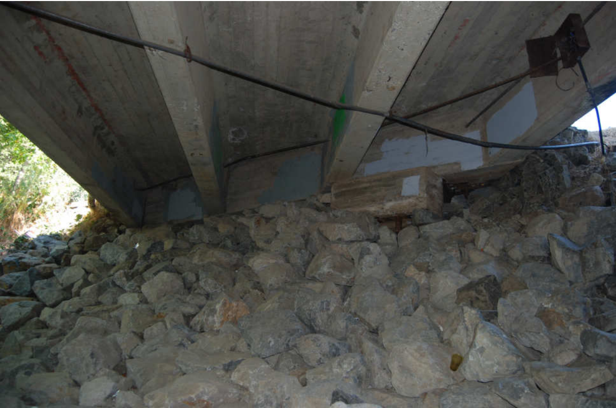
Finished riprap placement at Abutment 1
