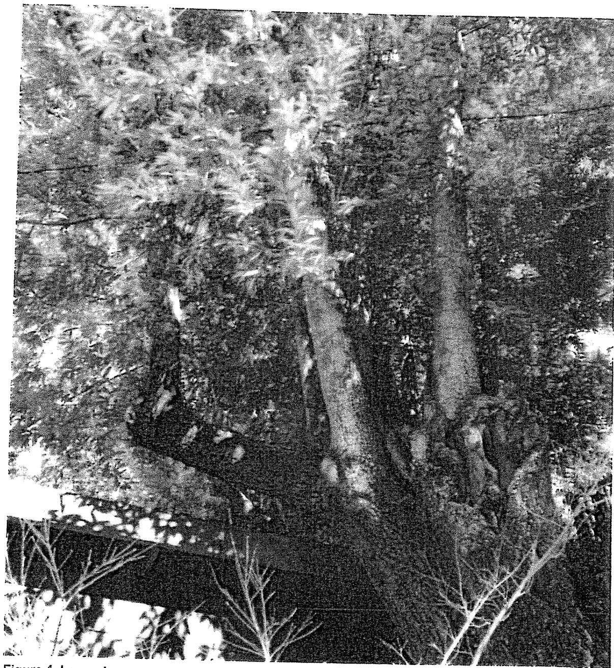
Figure 4. Large decay cavity at the common attachment point of all the major spars in Tree 1
