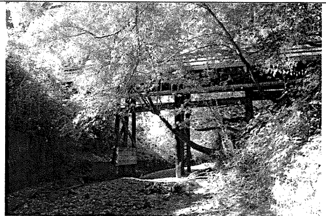
Photo 2: San Anselmo Creek beneath Meadow Way Bridge, August 2010.
