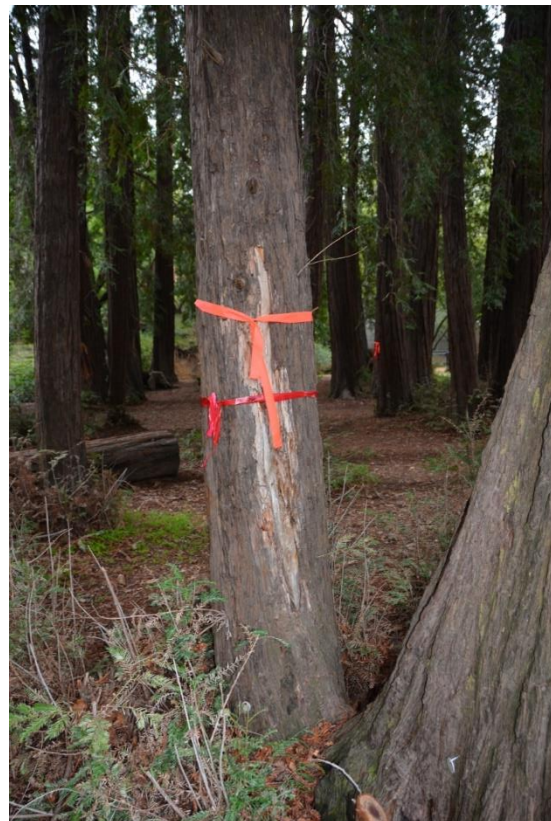
Figure 7 – This hollow tree has assumed a serious lean and the sap wood has died.
