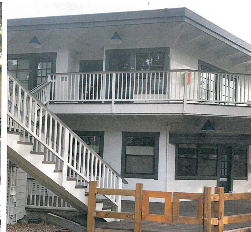
Existing Building Colors
