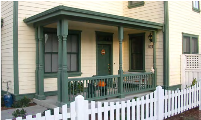
Example of an Engaged Porch
