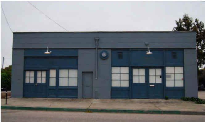
Example of a Maker Shopfront
