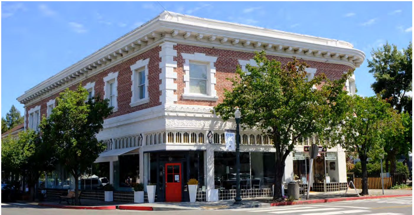
Example of Main Street Building
