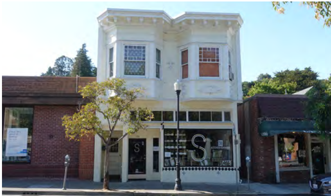
Example of Main Street Building
