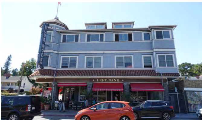
Example of Main Street Building
