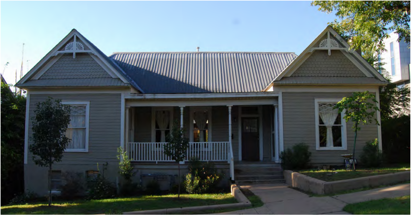
Example of an Engaged Porch
