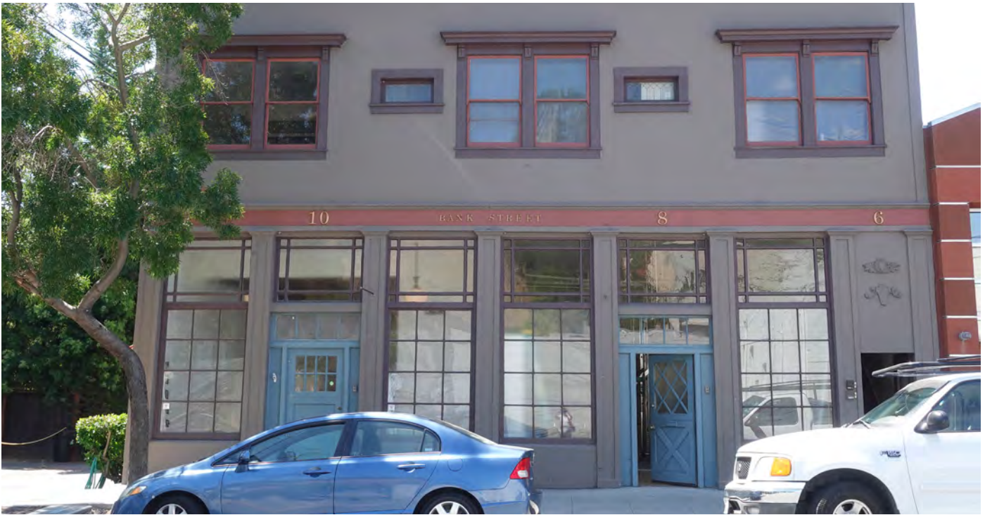
Example of a Maker Shopfront
