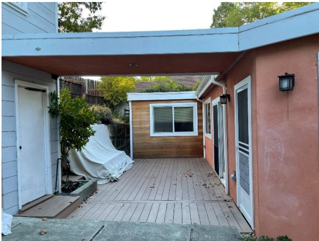
Covered Walkway before Removal
