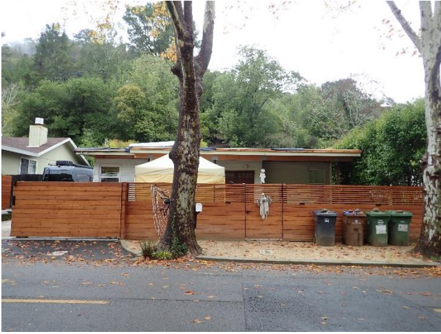
Front of House with New Eaves
