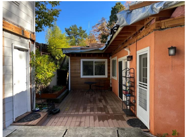
Area of Covered Walkway after Removal
