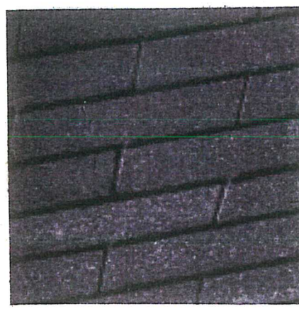
BLACK ASPHALT SHINGLE ROOF
