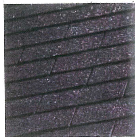
BLACK ASPHALT SHINGLE ROOF
