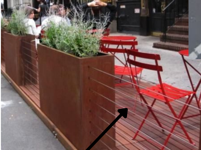
Metal Cable Railing
