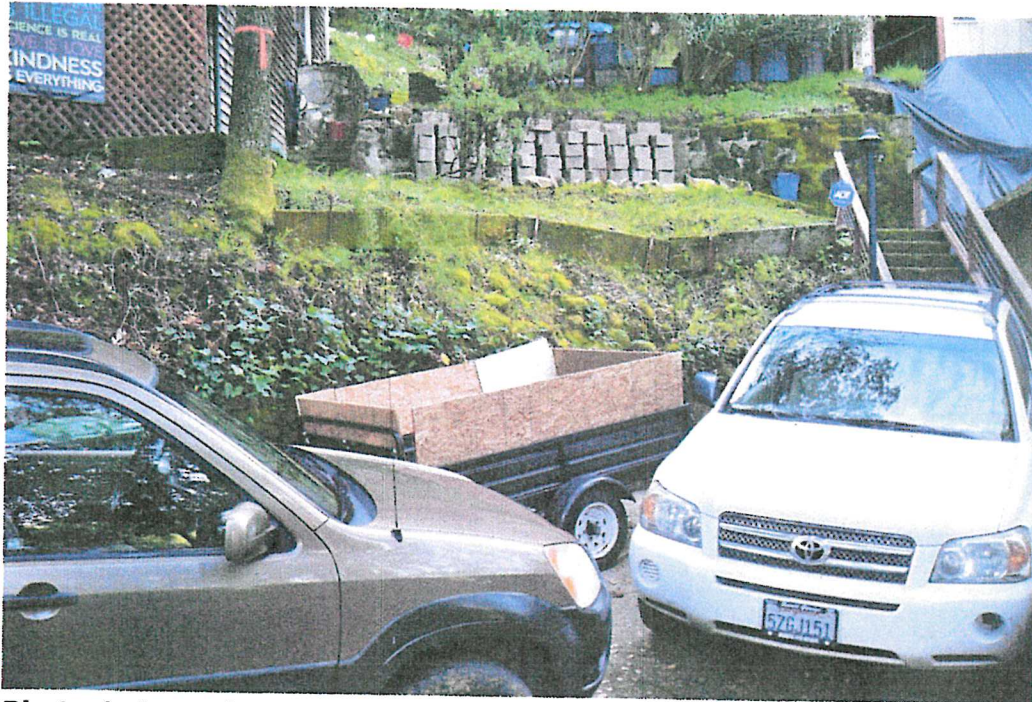
Photo 1. Area of proposed garage, looking southwest (uphill). The garage will be constructed between the house seen on the left and the boundary with the neighboring property on the right.
