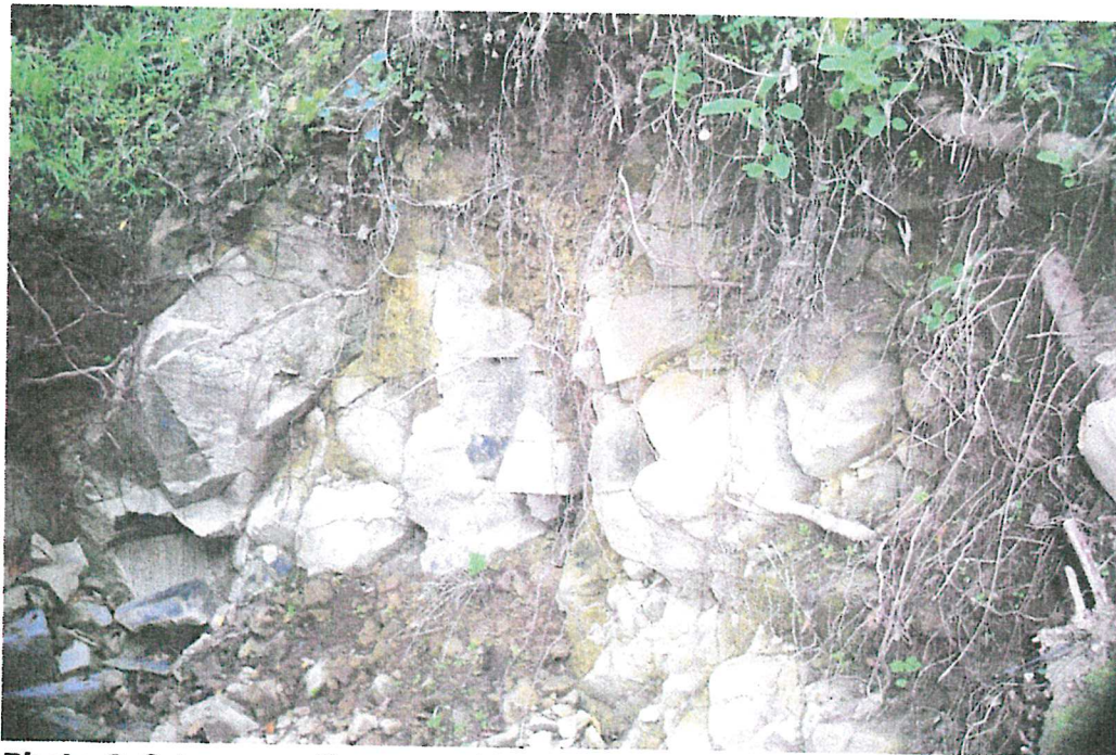
Photo 2. Cut near south corner of house, exposing bedrock, viewed looking southeast.
